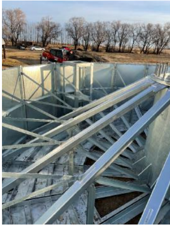
Bolts Torqued and Double Nuted
