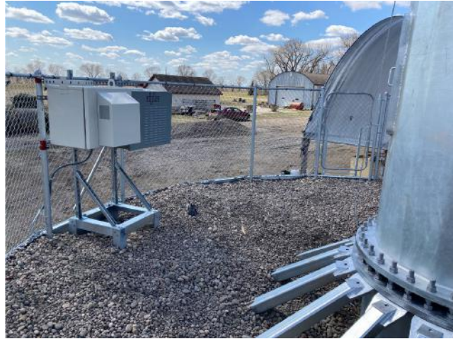
Ladders, Fencing, Cabinet Pedestals Added
