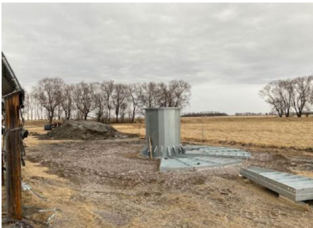
Base Pad Levelled, Kingpost and Outer Trays Set
