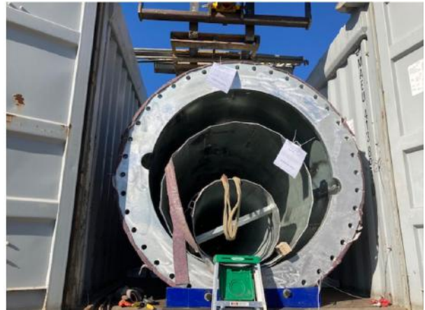
Off-Loading Pole Sections
