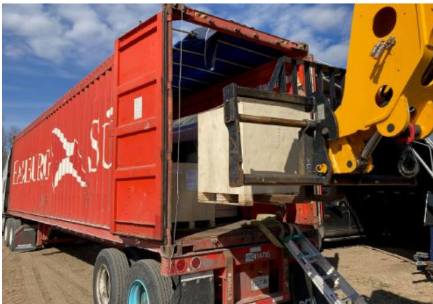
Off-Loading Foundation, Bolts, Antenna Mounts
