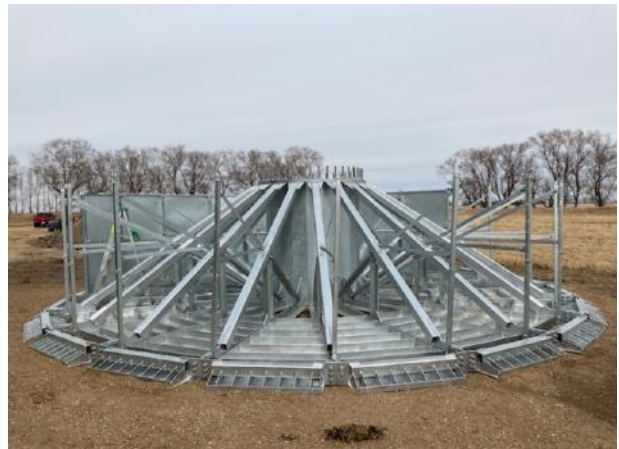
Truss Arms, Outer Trays and Side-Walls Added
