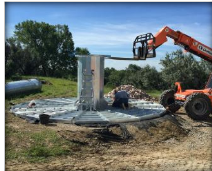
Assembly of the base trays
