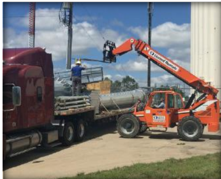
Off-loading flatbed truck
