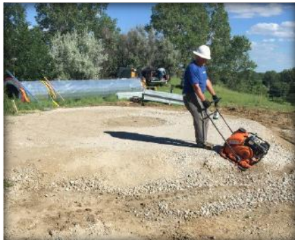
Preparing compacted gravel base
