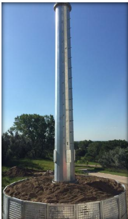
Foundation with 1 st pole section
