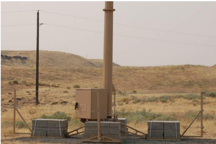
Foundation with ballast completed
