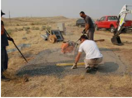
Leveling the base
