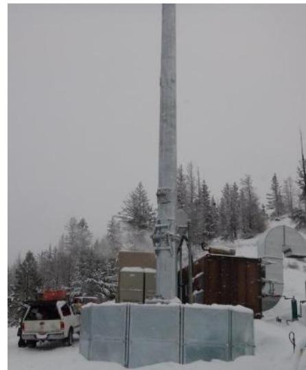
AFS 1100 foundation & 60' self-raising pole installed
