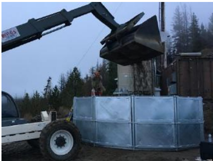
Foundation filled with ballast
