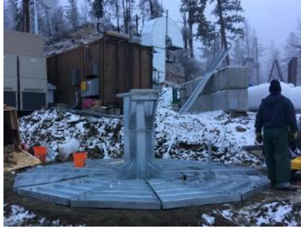
Site leveled on mountain top & preassembly of the base
