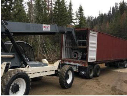
Pole and foundation off-loaded at the base of the mountain
