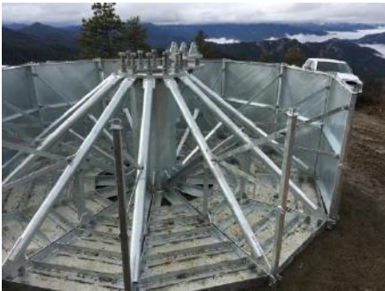
Foundation side wall assembly
