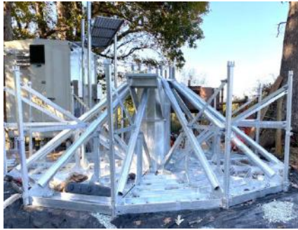
Foundation with truss arms
