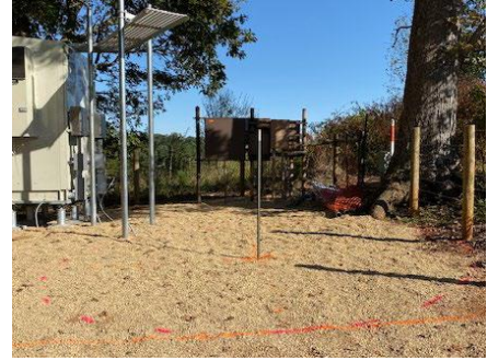
Very limited space to install the foundation
