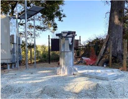
Leveled foundation pad with kingpost
