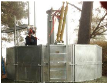
Foundation and hydraulic rams
