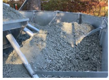
Foundation with ballast
