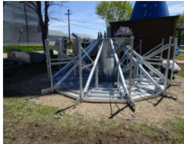
All truss arms assembled
