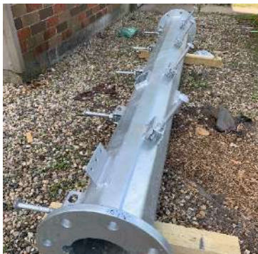
Ballast added – Pole assembled
