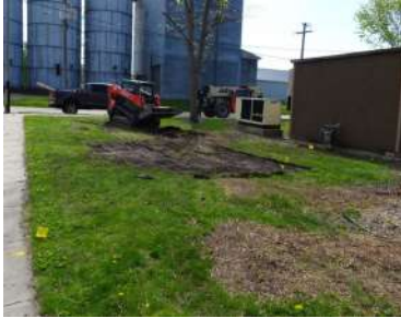
Top sod removed
