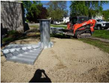
Kingpost and base trays laid out
