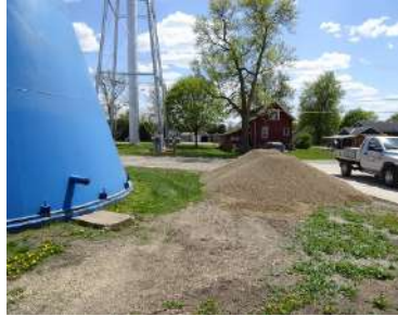
Gravel/Rock/Class 5 for ballast & pad
