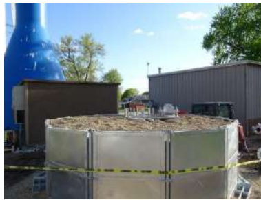
Ballast added – Pole assembled
