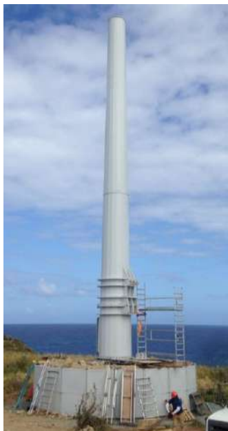
AFS 2000 foundation & 22m tilt-up pole installed
