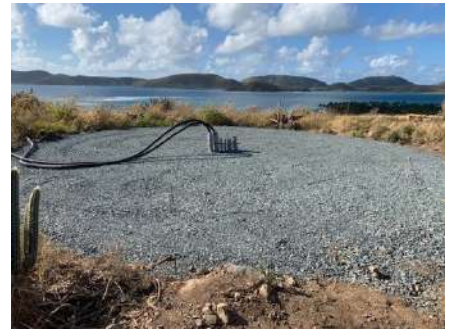
Leveled base with electrical to center
