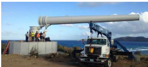
Installed tilt-up pole
