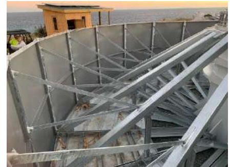
Fully assembled foundation
