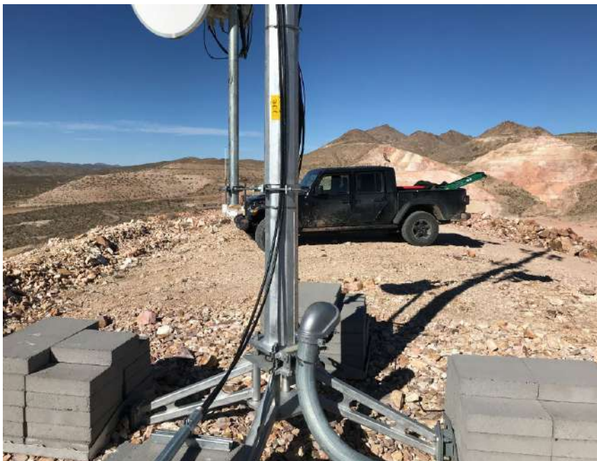
Electrical and RA Work Completed
