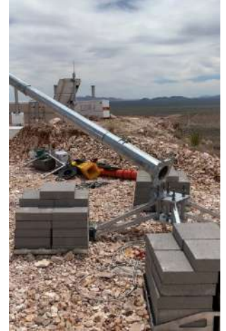
Tilt-up Pole, Level & Nut
