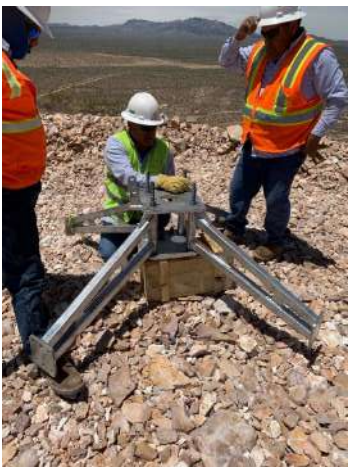
Assemble Plates Hub & Legs
