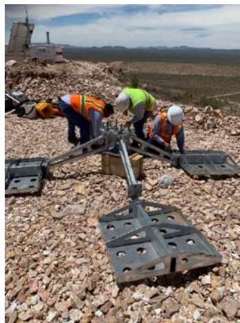
Add Outer Trays and Ballast
