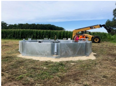
Ballast Tanks Set and Filled
