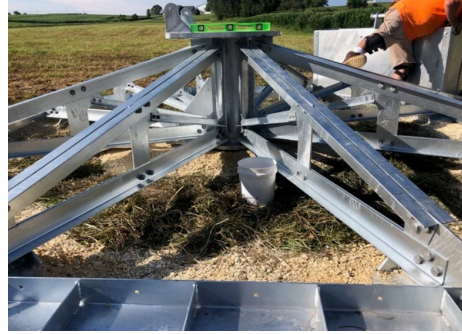
Level Area, Assemble Truss Arms/Trays
