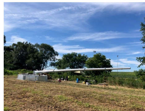
Pole Built, Climbing Pegs/Mounts Added
