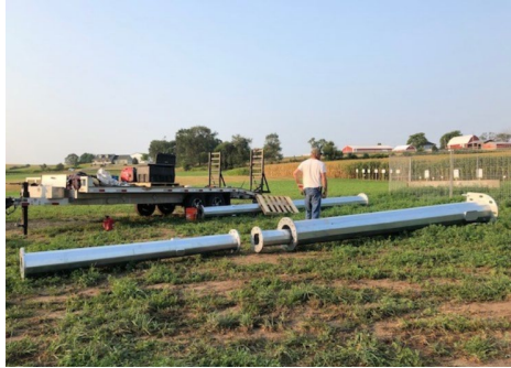
Pole and Foundation Off-Loaded
