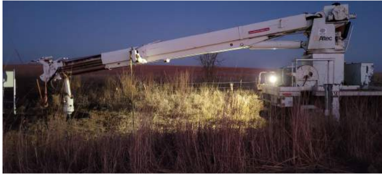
Step 2 & 3: Base Pole Section Set in Hole and Shimmed, Expanding Foamed Added
