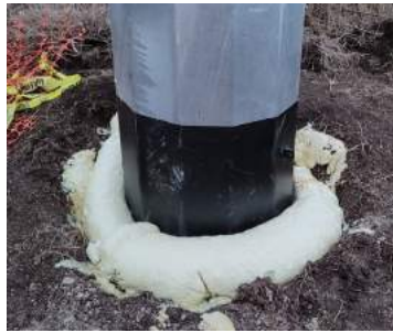
Step 2 & 3: Base Pole Section Set in Hole and Shimmed, Expanding Foamed Added
