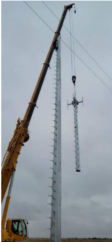
Step 4: Assembly of Slip-Jointed Pole
