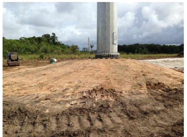
Foundation Backfilled and Ready for Turbine
