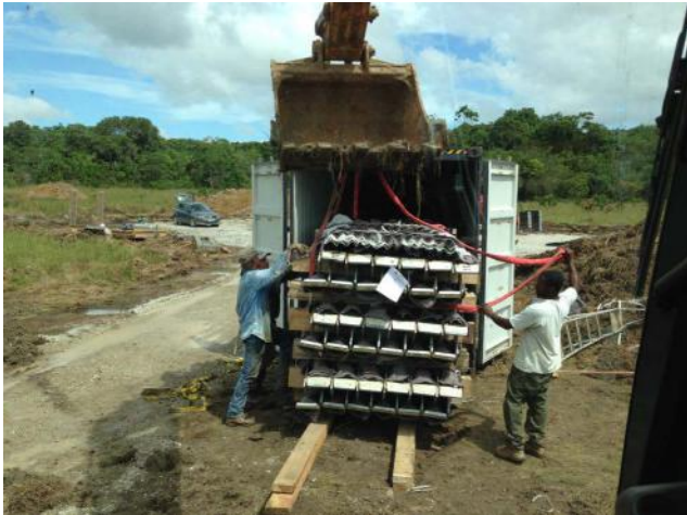
Unloading the Foundation
