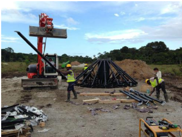
Setting the Foundation Stringers
