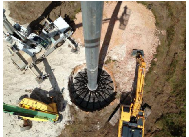
Foundation Placed and Tower Attached
