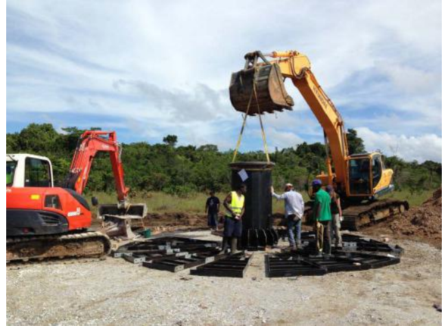
Setting the Foundation King Post
