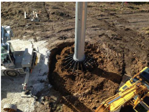
Backfilling and Compacting Local Soils
