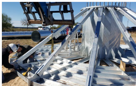
Truss arm assembly
