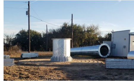
Kingpost on leveled pad
