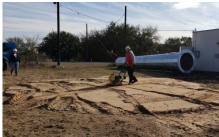
Preparing pad for foundation
