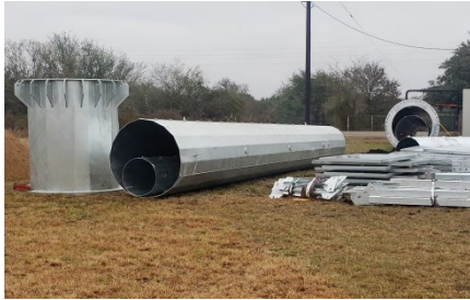
AFS and pole sections off-loaded at site
