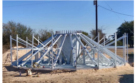
Truss arm assembly
