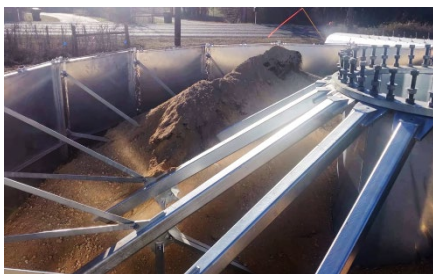
Foundation filled with ballast
