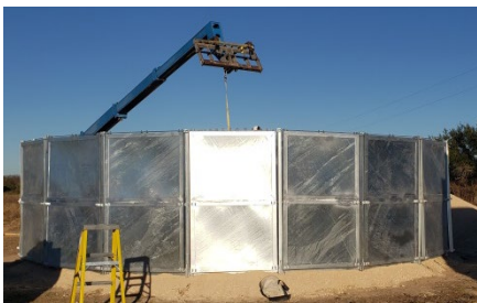
Fully assembled foundation
