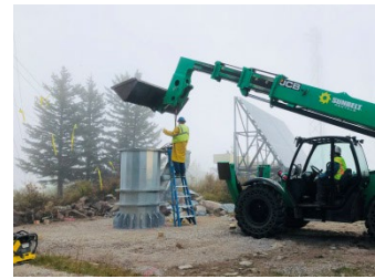
Pad completed and Kingpost set
