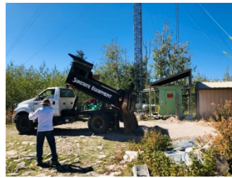
Preparing pad for foundation
