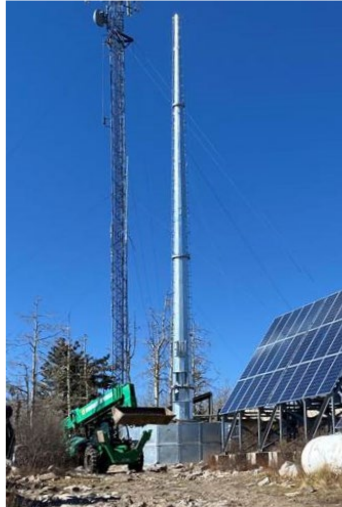
AFS 1700 foundation & 85' pole installed
