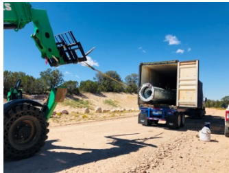
AFS foundation and pole arrive in a container
