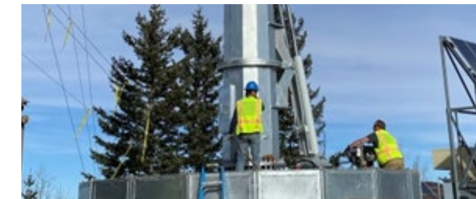
Pole raised with ARE hydraulic system
