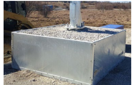
Foundation with ballast
