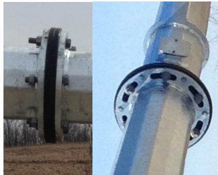
Customized aluminum plate allowing for precise positioning of the antenna
