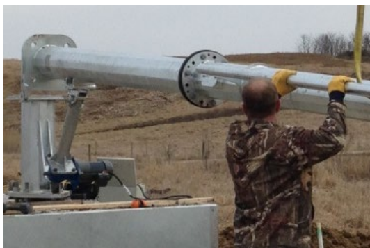
Customized aluminum plate allowing for precise positioning of the antenna
