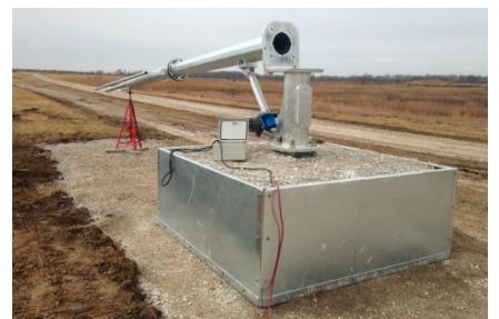
Motorized screw jack to raise the pole
