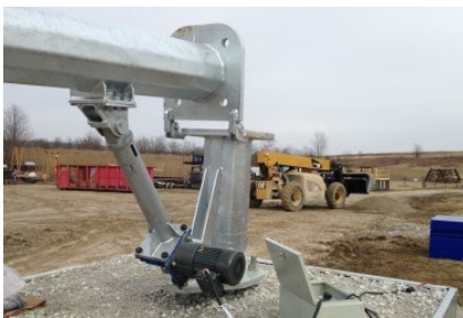
Motorized screw jack to raise the pole
