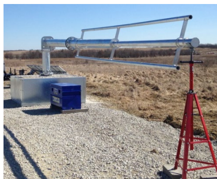
Install AFS 350 and pole
