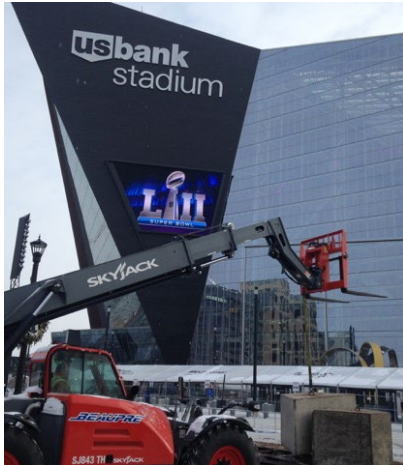
Concrete blocks for ballast
