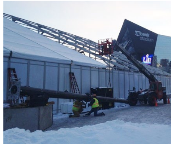
Foundation with ballast concrete blocks
