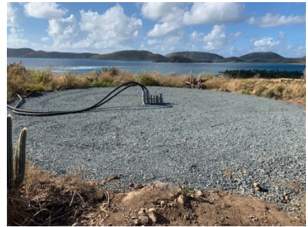
Leveled base with electrical to center
