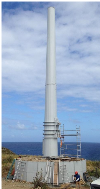
AFS 2000 foundation & 22m tilt-up pole installed
