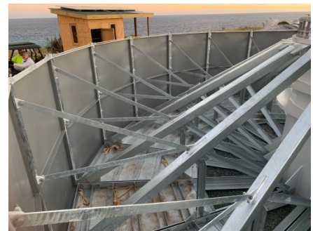
Fully Assembled Foundation
