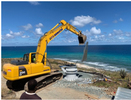
Track-hoe only equipment used
