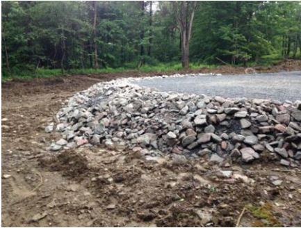
Leveling installation site
