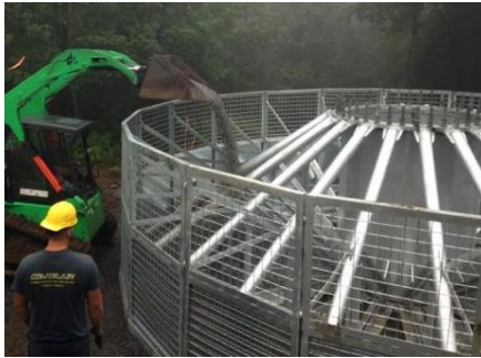
AFS with sidewalls filled with ballast
