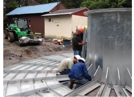
Preassembly of the base
