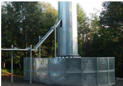
AFS 1900 foundation & 100' flanged pole installed
