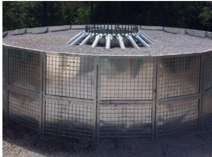
Foundation with ballast
