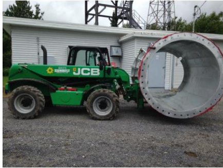
King post moved to installation site
