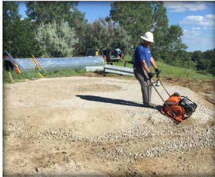
Preparing compacted gravel base
