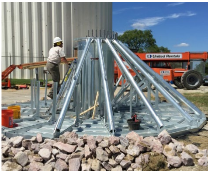
Assembly of the support arms
