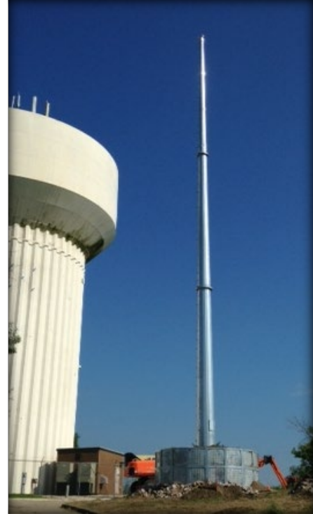
AFS 1500 foundation & 100' pole installed supporting 2-3 carriers
