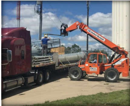
Off-loading flatbed truck
