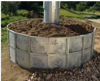
Foundation with ballast
