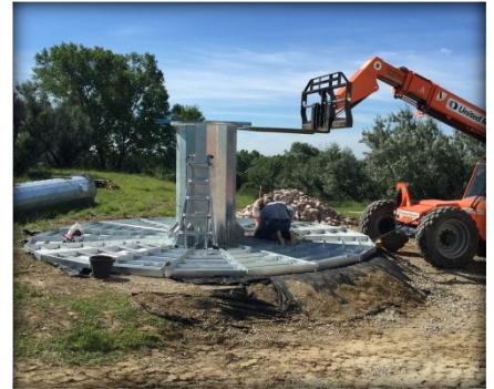
Assembly of the base trays
