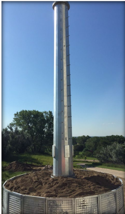
Foundation with 1 st pole section
