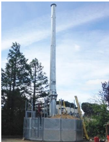
Foundation with ballast and pole
