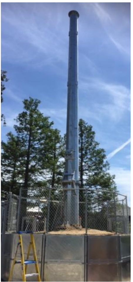
AFS 1100 foundation & self-raising pole installed
