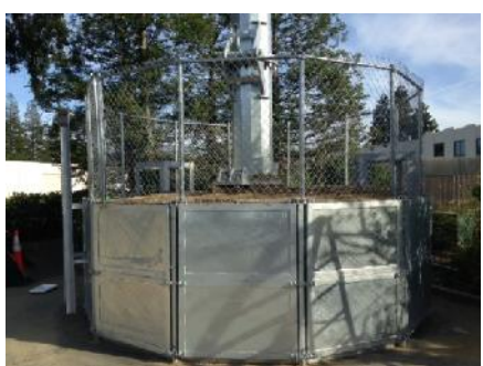
Foundation with fencing and ladder
