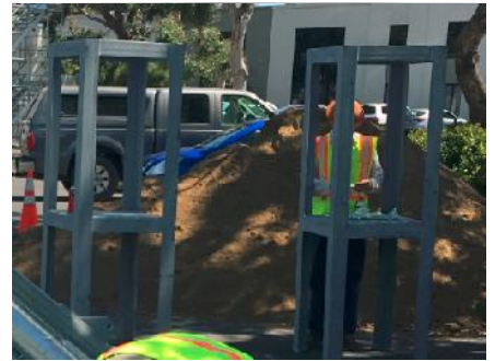
Cabinet holders to be installed inside the foundation
