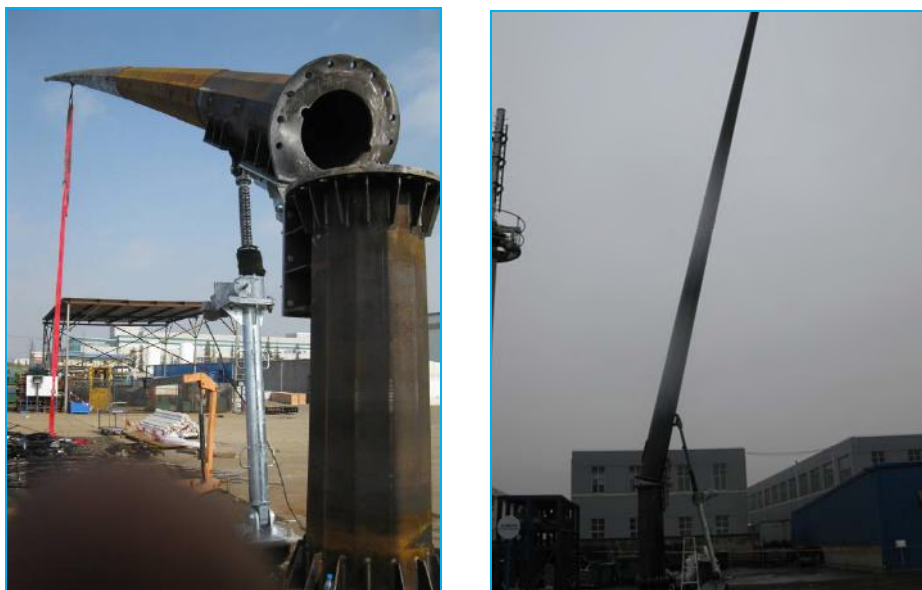
Figure 20 Raising the pole
