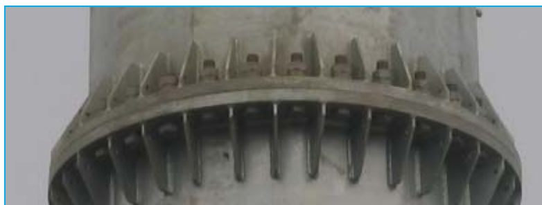
Figure 20 Fix section B to the section A using all bolt
