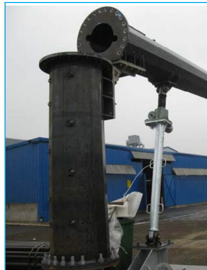
Figure 17 Fix the top of Mechanical Jacking Device to section B
