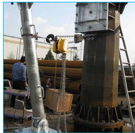
Figure 10 Lift the Mechanical Device
