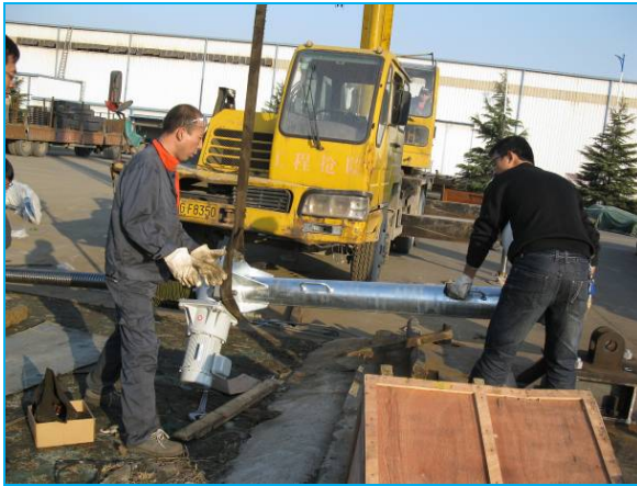
Figure 9 Lift the worm screw
