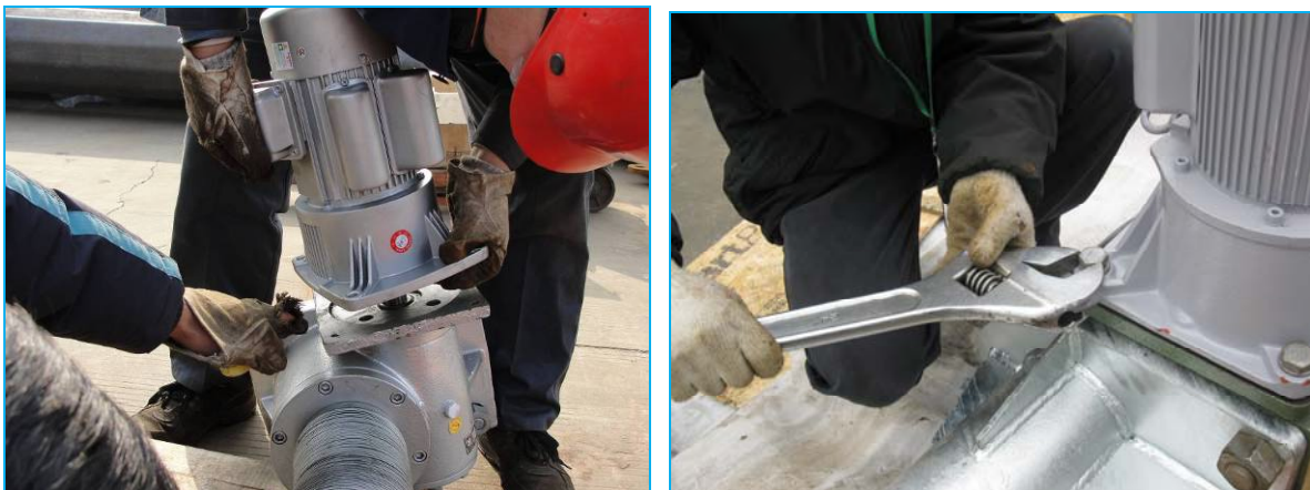
Figure 8 Install the motor
