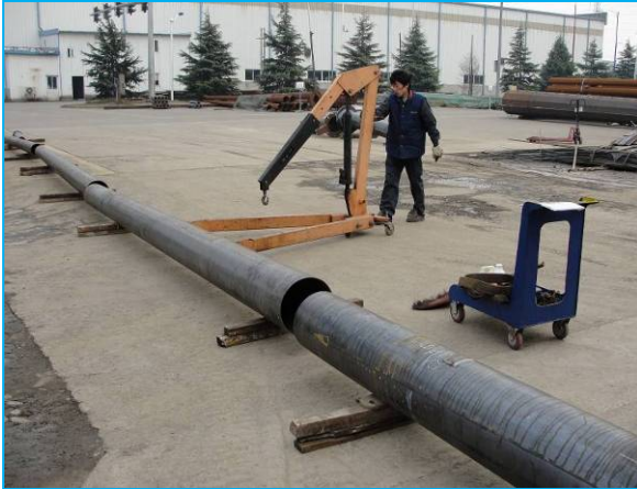
Figure 1 Align all sections
