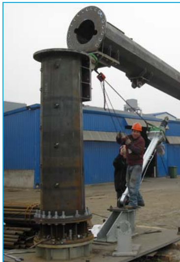
Figure 17 Fix the top of Mechanical Jacking Device to section B
