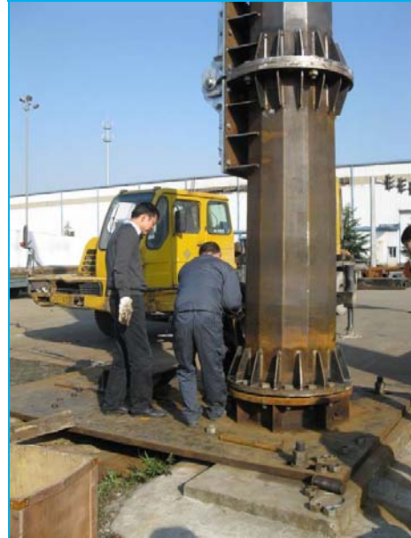
Figure 6 fix the base section
