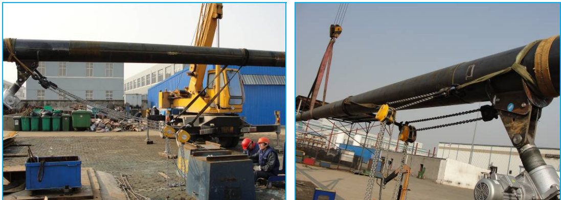
Figure 19 Secure the section B and other sections tightly
