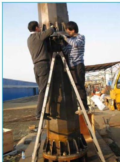
Figure 16 Remove the bolts
