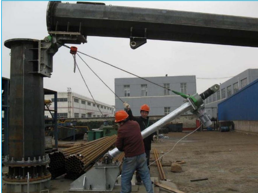
Figure 17 Rotate section B to horizontal position
