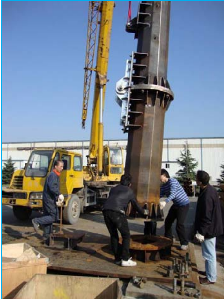
Figure 5 Lift the base section
