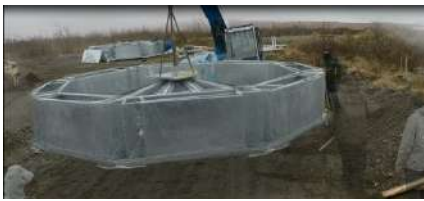
Foundation moved to site
