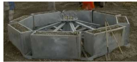
Foundation with ballast tank filled with dirt
