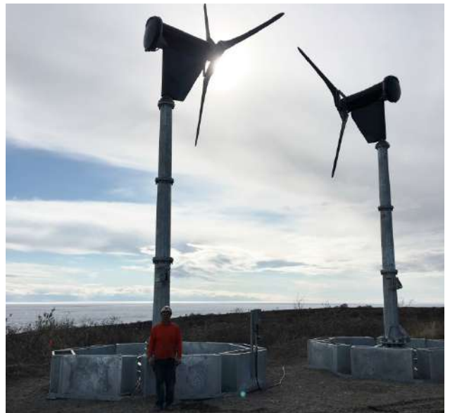
AFS 550 foundations & 30' self-raising poles installed
