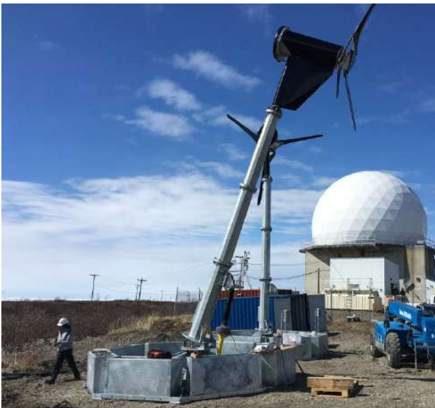
AFS 550 foundations & 30' self-raising poles installed
