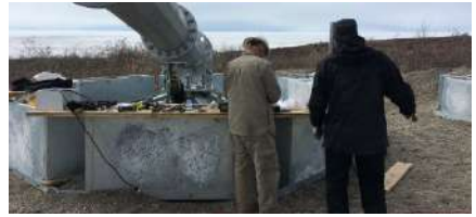
Tower raised with screw jack
