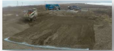
Prep site with styrofoam for permafrost
