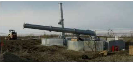
Tower raised with screw jack
