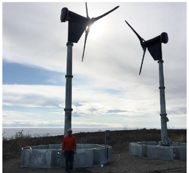
AFS 550 foundations & 30' self-raising poles installed
