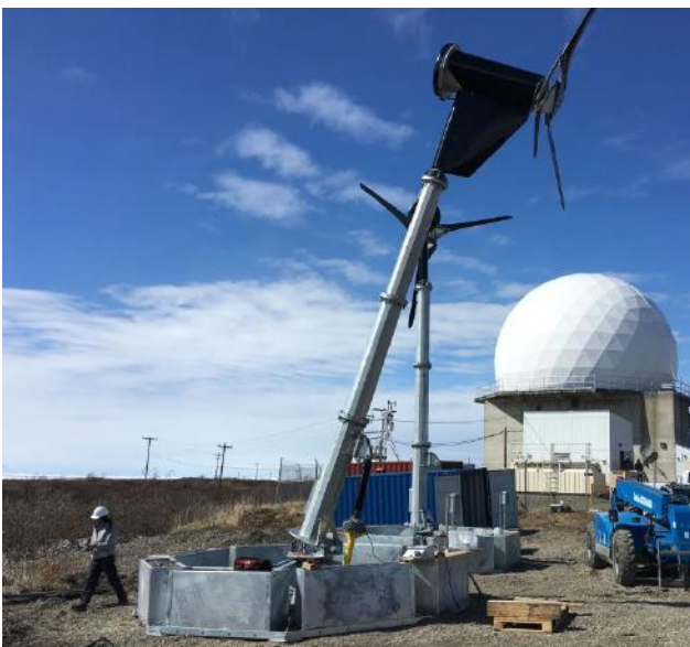
AFS 550 foundations & 30' self-raising poles installed
