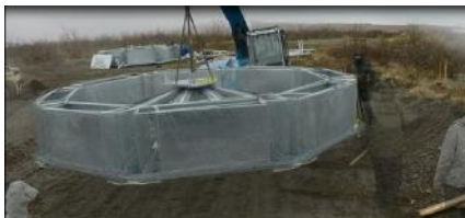
Foundation moved to site
