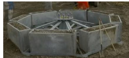
Foundation with ballast tank filled with dirt
