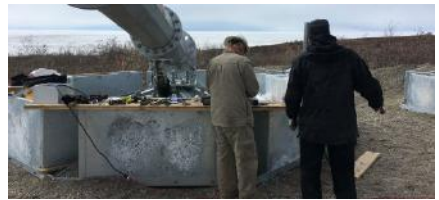
Tower raised with screw jack
