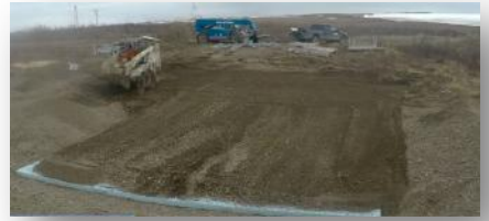
Prep site with styrofoam for permafrost
