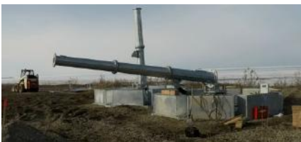
Tower raised with screw jack
