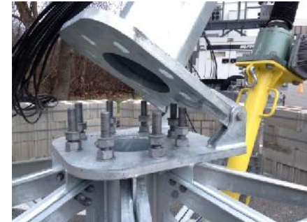
Motorized screw jack raising pole
