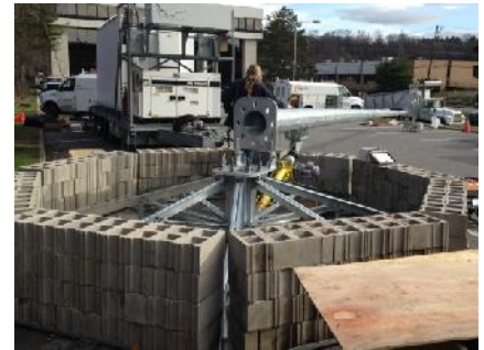
Installation of antennas
