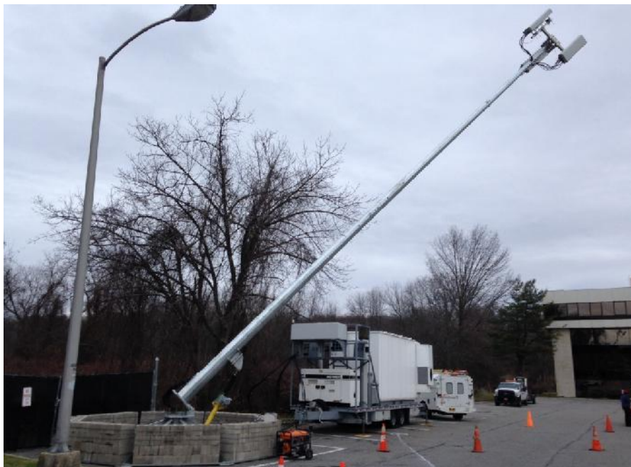
AFS 500 foundation & 60' self-raising pole installed
