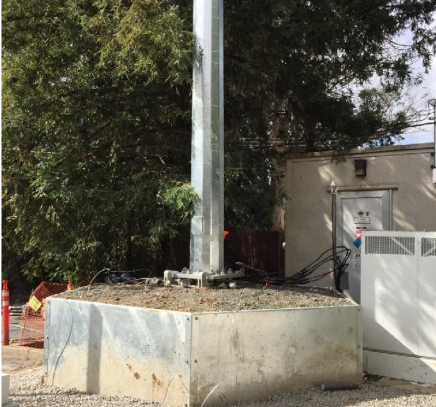
Foundation filled with ballast
