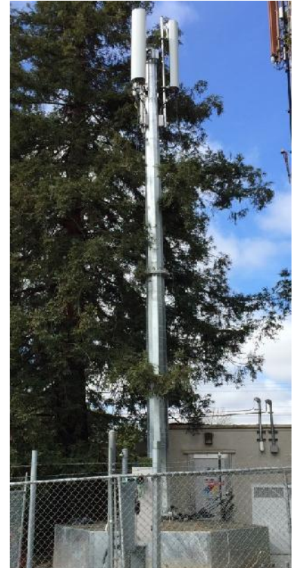
Foundation & 36' self-raising pole
