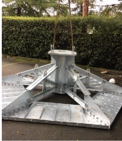
Assembly of the base
