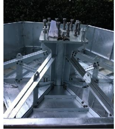
Foundation with sidewalls
