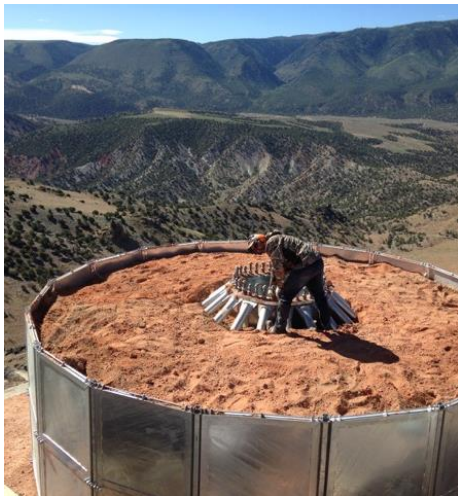
Foundation with ballast completed
