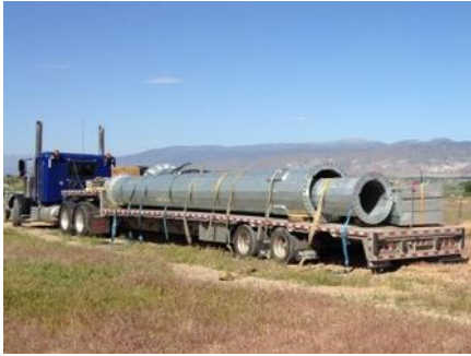
Delivery of the foundation and pole at the base of the mountain
