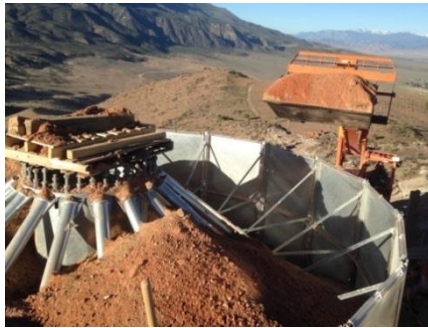
Foundation with sidewalls and filled with ballast
