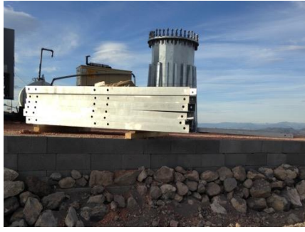
Parts brought to the mountain top with a forklift and assembled on a leveled area
