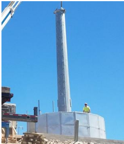
Foundation with pole (1 st section)
