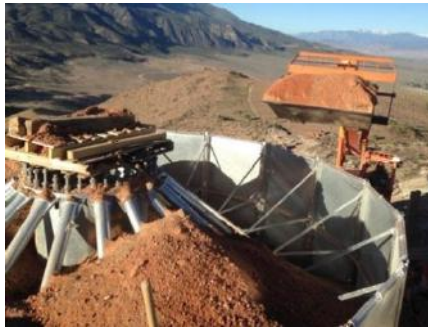
Foundation with sidewalls and filled with ballast
