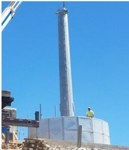
Foundation with pole (1 st section)
