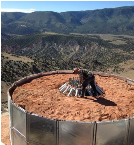
Foundation with ballast completed
