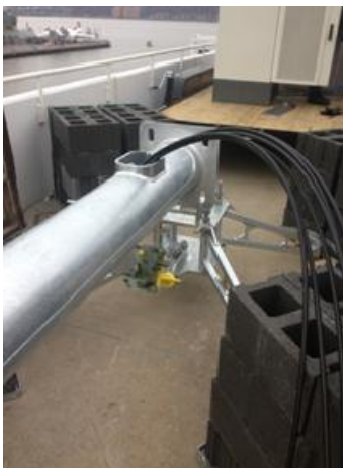
Telecom Equipment Install
