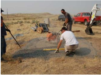
Leveling the base
