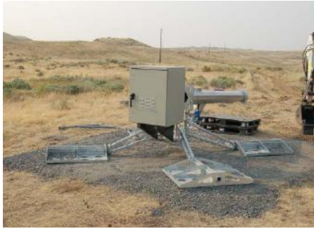
Assembled Foundation with electrical box
