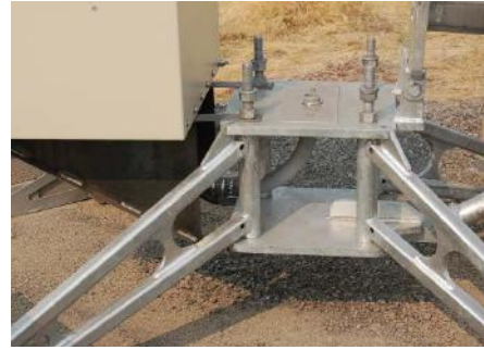
Assembled Foundation with electrical box
