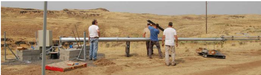
Foundation with ballast and pole. Solar panel and antenna assembly.
