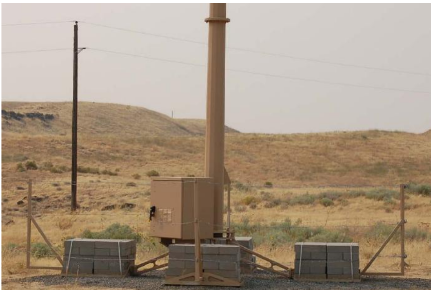
Foundation with ballast completed
