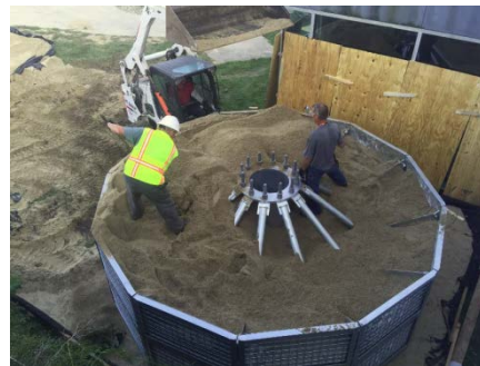
Foundation with ballast
