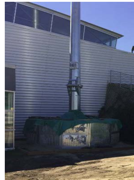
Self-raising slip joint pole assembly
