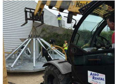
Foundation moved to site
