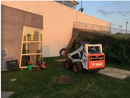
Leveling installation site
