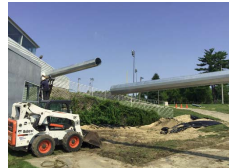
Self-raising slip joint pole assembly
