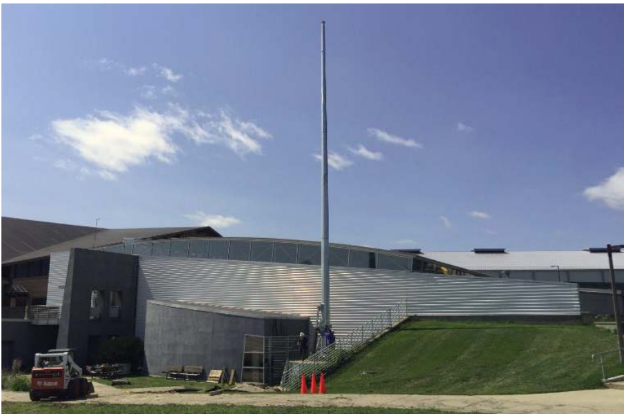
AFS 1100 foundation & 80' self-raising pole installed
