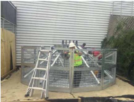
Foundation side walls assembly
