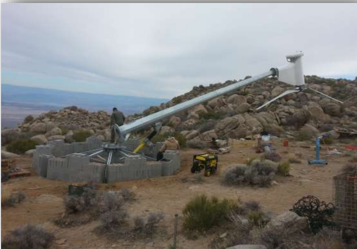
Tower with Kingspan 6kW turbine is ready to be raised with our 25 ton tower raising system.
