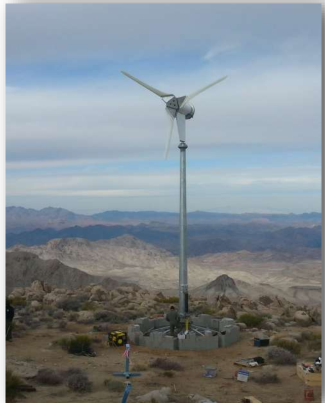
Tower System with turbine attached raised into position.
