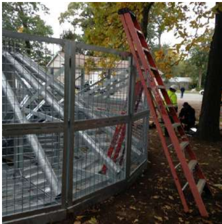
Side Walls Installed
