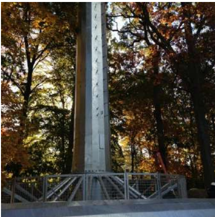
Foundation and First Pole Section Set Prior to Ballast Fill
