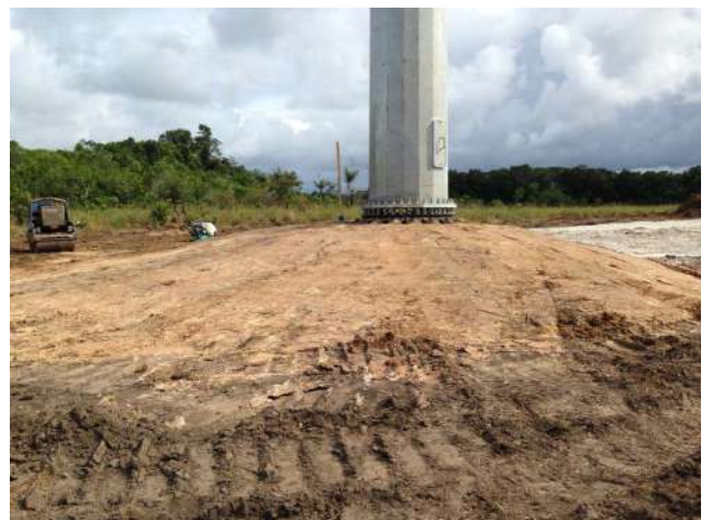
Foundation Backfilled and Ready for Turbine
