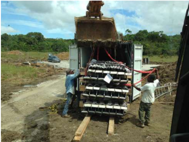
Unloading the Foundation
