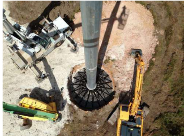
Foundation Placed and Tower Attached
