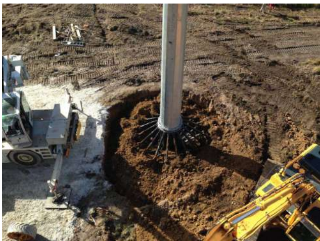
Backfilling and Compacting Local Soils
