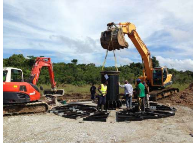
Setting the Foundation King Post
