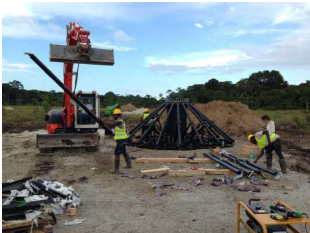
Setting the Foundation Stringers
