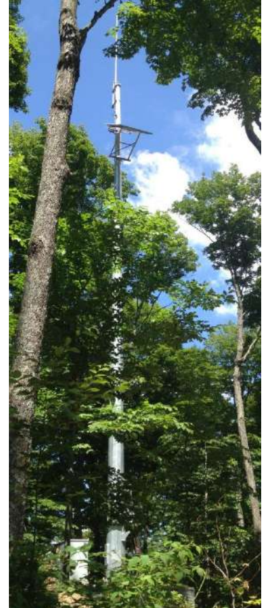
Foundation & 80' pole installed
