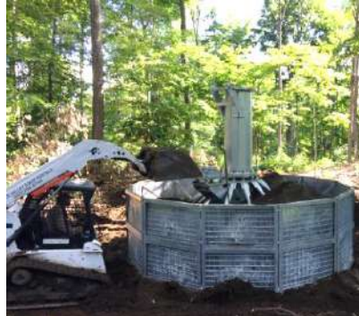
First pole section installed as ballast is completed
