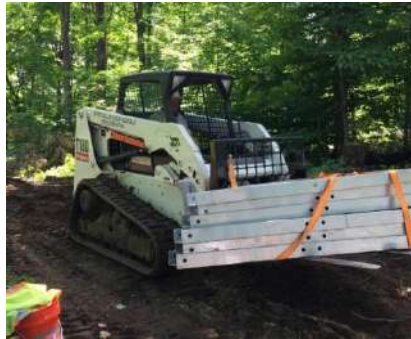
Foundation hauled to mountain top
