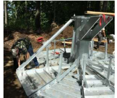
Installation of base trays and support arms
