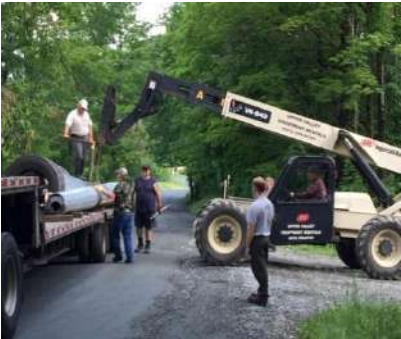
Off-loading flatbed truck
