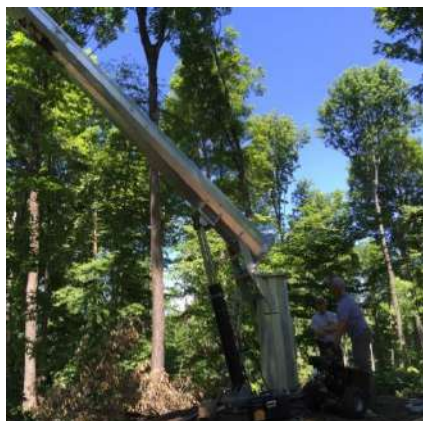
Pole raised using hydraulic rams
