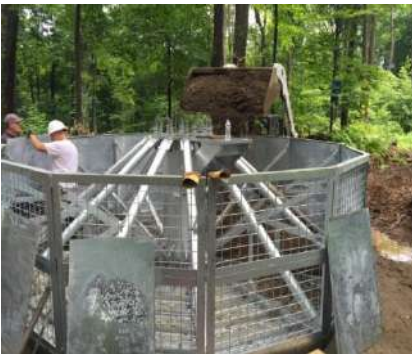
Installing side-walls while ballast is added
