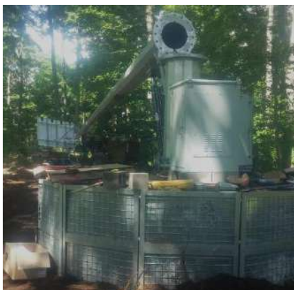
Pole and solar panels assembled
