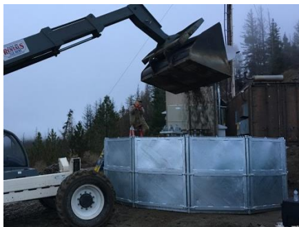
Foundation filled with ballast
