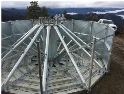
Foundation side wall assembly
