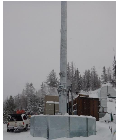
AFS 1100 foundation & 60' self-raising pole installed
