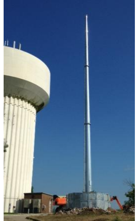
AFS 1500 foundation & 100' pole installed
