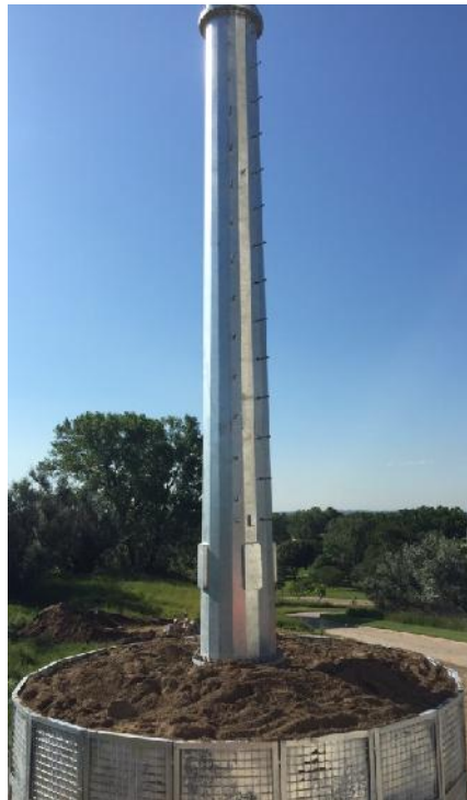
Foundation with 1 st pole section
