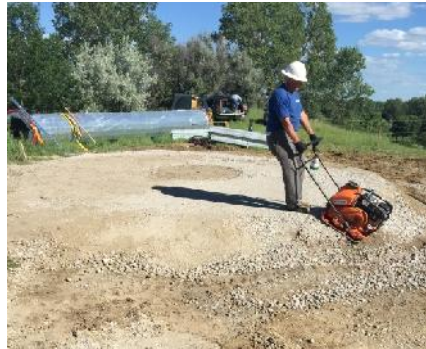
Preparing compacted gravel base
