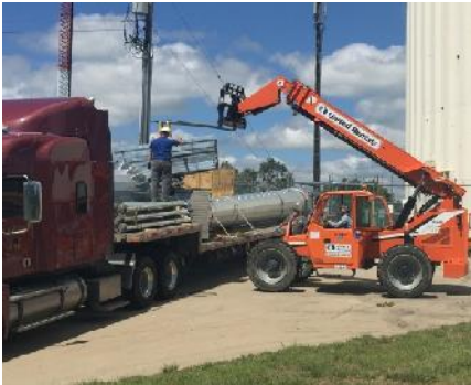
Off-loading flatbed truck
