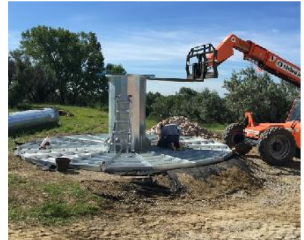
Assembly of the base trays
