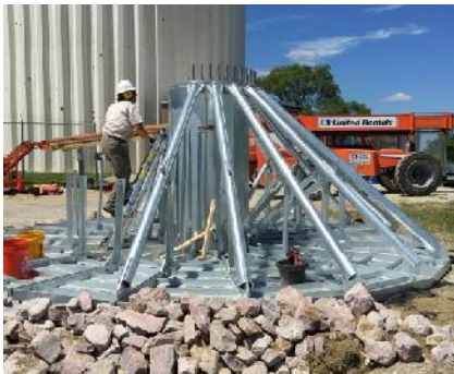
Assembly of the support arms
