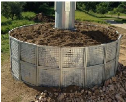
Foundation with ballast
